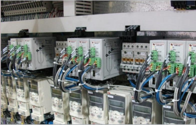
The Ultra-fast Techna-Check transducers are developed specifically for Machine Tool Monitoring applications and can monitor both AC and DC loads. These sensors mount in the electrical cabinet of the machine and communicate with the Techna-Check units using the proprietary TTBUS network.
